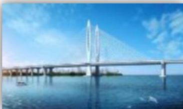
江西吉水赣江二桥 2014 Ganjiang No.2 Bridge
