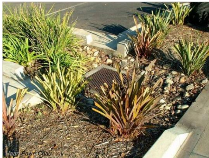
Curb cuts leading to an infiltration zone at the Rio Hondo Golf Course in Downey, CA
